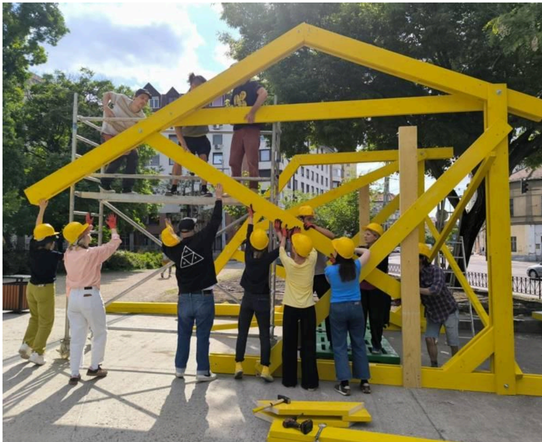
AllinOne – construction work at Kálvária Square, April 28 – May 10, 2025. Photo: Santiago Cirugeda.
